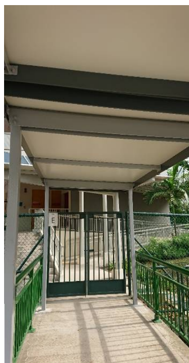
Shelter to school's Gate E
